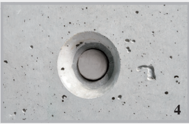
Flush seal for distance tubes with cone.
