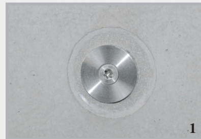
Sealing of distance tube with lip.
