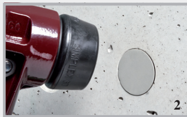
Drive in with rubber mallet
