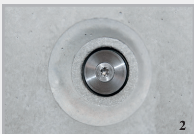
Flush seal for distance tubes with cone.
