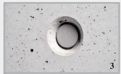
Sealing of distance tube with cone
