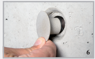
After inserting the STOPPER in, a cone can be glued in.
