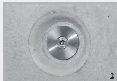
Sealing of distance tube with cone.
