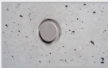
Sealing of distance tube with lip
